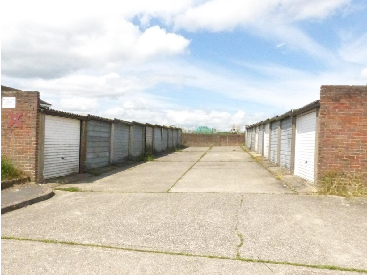
Martlett Road Garages 1-23
